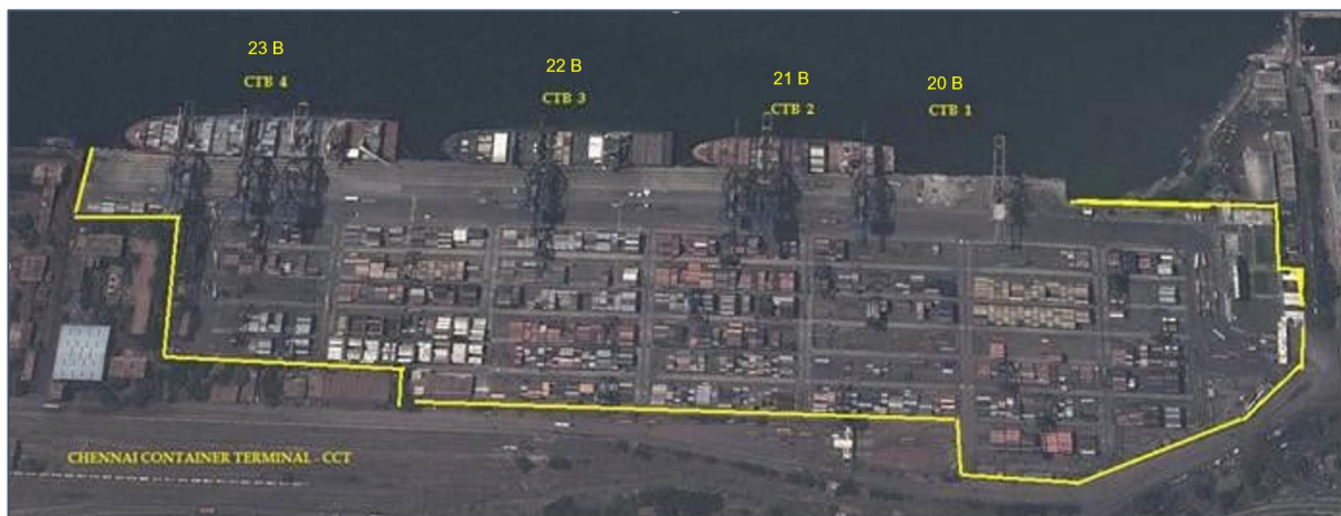
Figure 3-4: Container Terminal in the Bharathi Dock
