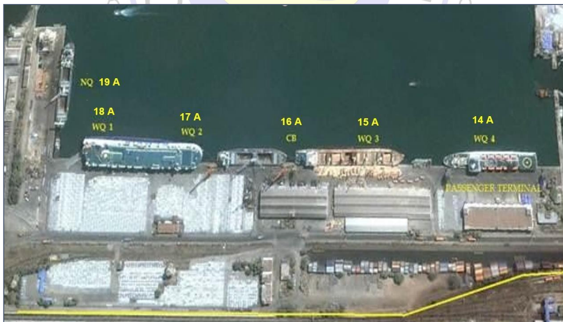
Figure 6.9: North Quay and West Quay Berths
