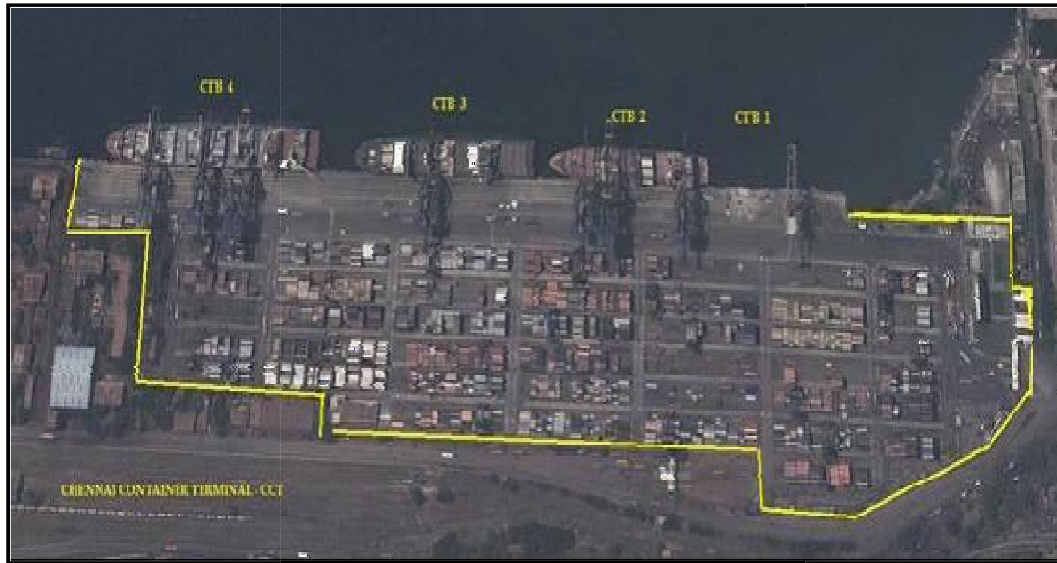
Figure 6.5 Chennai Container Terminal (CCTPL)
